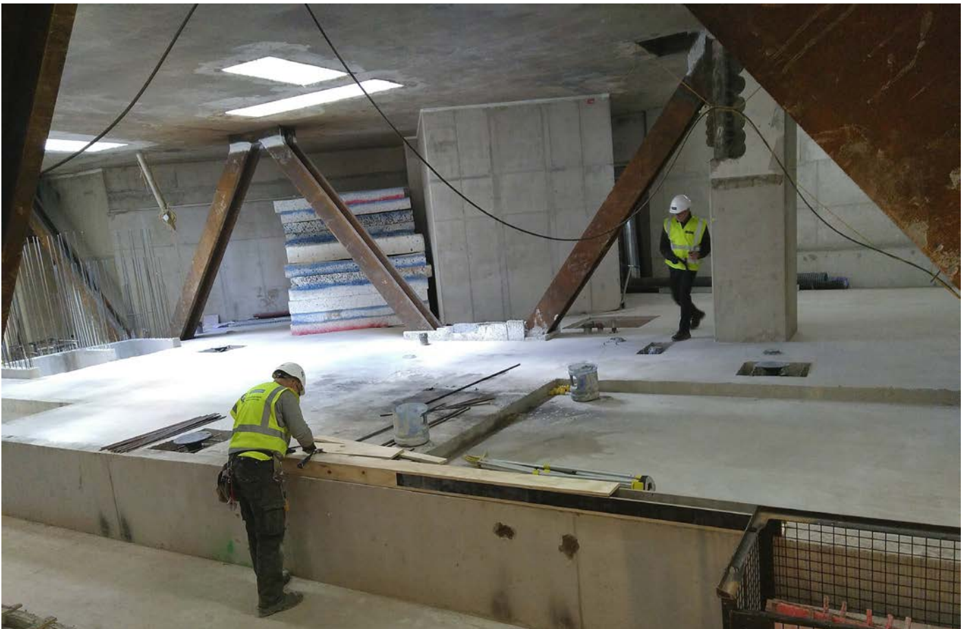
above: 1 Soho Place steel core in construction below: Transfer trusses within 4 Soho Place basement
