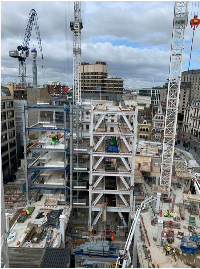
above: 1 Soho Place steel core in construction below: Transfer trusses within 4 Soho Place basement
