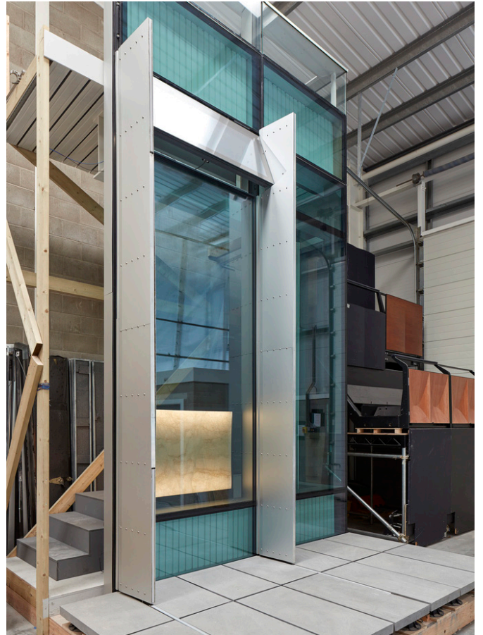
above: Site B back of house benchmark below: Site B office facade - confirming fin depth and backbox geometry
