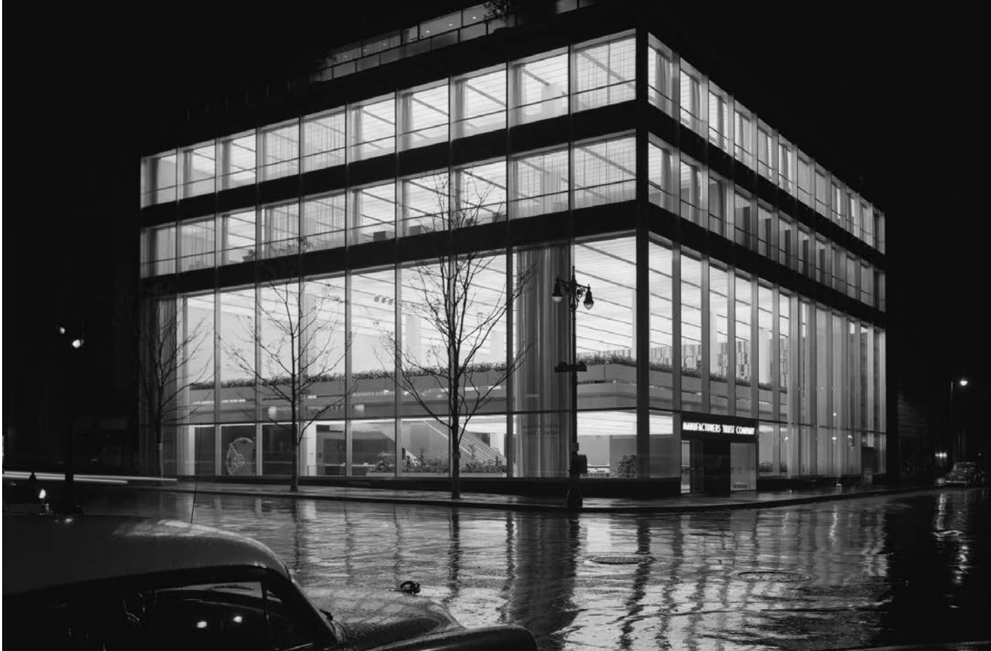
Manufacturer's Trust Building, New York Charles Evans Hughes III and Gordon Bunshaft of Skidmore, Owings & Merrill (SOM). Completed 1954
